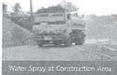
Water Spray at Construction Area
